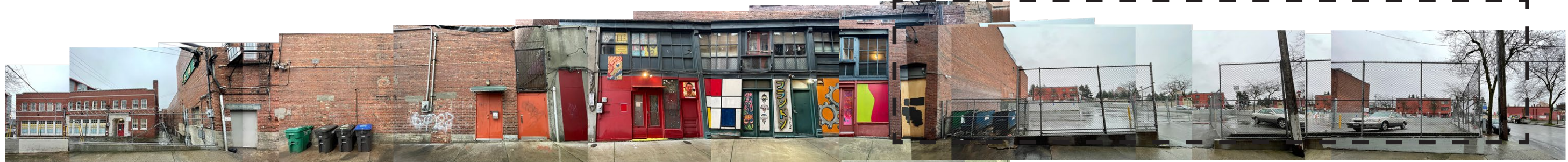
▶ North Block, Facing West
