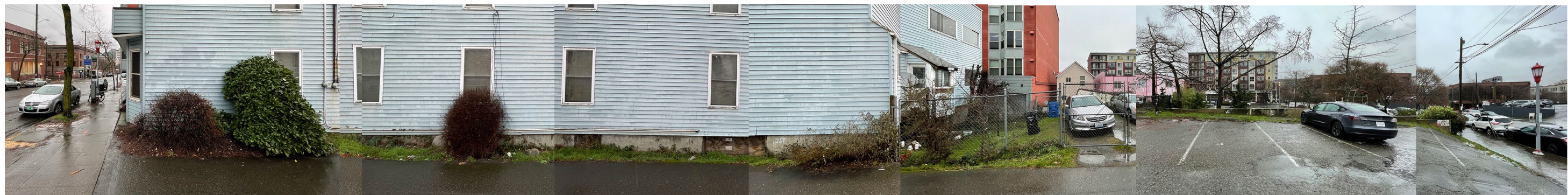
▶ South Block, Facing East
