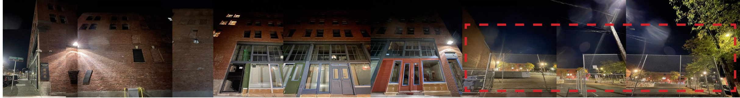
▶ North Block, Facing East
