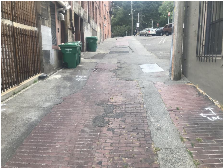
Plate 4. Middle portion of Nihonmachi Alley, looking north
